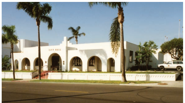
The Oceanside City Hall building, now the home of the Oceanside Museum of Art, its a great example of Gill's work.
